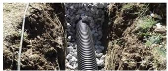
A simple French Drain is a trench or hole filled with gravel that allows surface water to soak into the ground, alleviating standing water and providing more irrigation to nearby vegetation. A more sophisticated French Drain can use perforated pipes to direct water elsewhere and allow the water to slowly soak into the surrounding soil.
