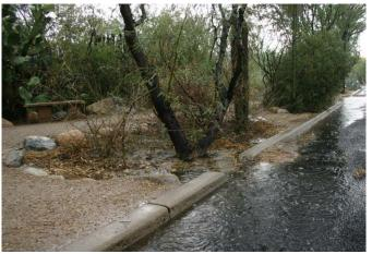
A curb cut is literally a cut in a street curb that allows storm water to flow from the street into a mulched basin, swale, or French Drain. Many neighborhoods in Tucson use curb cuts to move rainwater to community landscaping areas.
