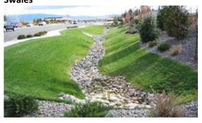
Swales are shallow ditches, usually perpendicular to the direction of water flow, that collect storm water and allow it to sink slowly and directly into soil. Their placement permits the redirection of water from its natural direction of flow to another desired location.
