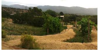
Berms are low mounds of earth formed to help hold water in basins or swales. Often the soil used to create a berm was excavated by digging a basin or swale.
