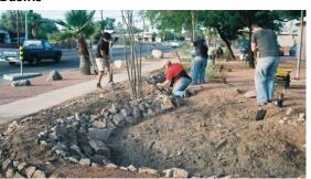
Basins are excavated shallow areas, often lined with rock or mulch that accept rainwater runoff and permit water to percolate into the soil. Basins connected by shallow, sloping (1/4 inch per 1 linear foot) swales allow water to flow from one basin to another.
